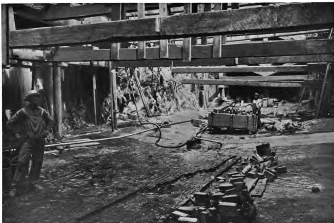
SPECIAL BRICK AND ASPHALT WATERPROOFING
